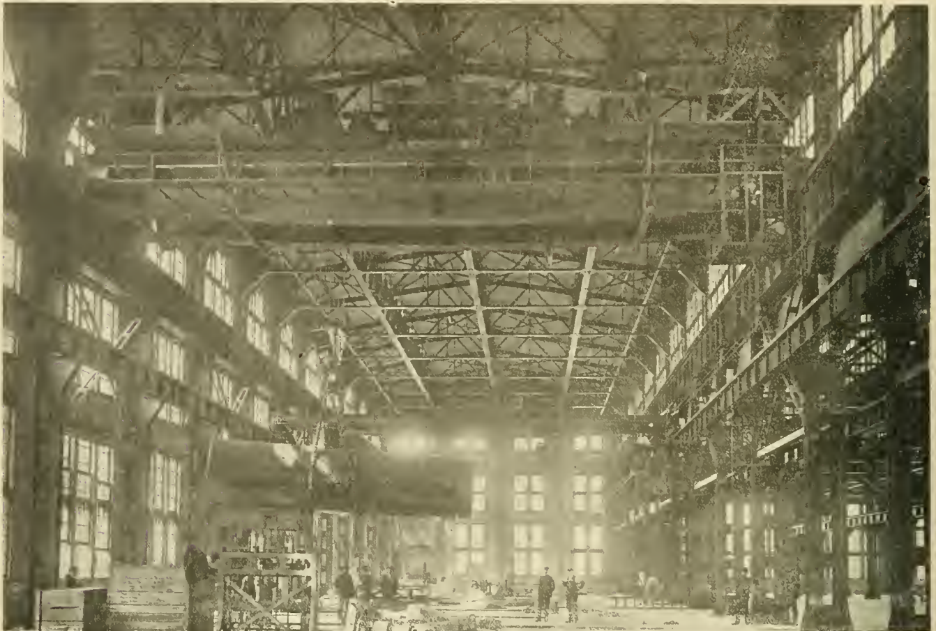
INTERIOR VIEW IN ERECTING SHOP, SHOWING 120-TON CRANE LIFTING A BOILER, SHOWING ALSO HEAVY CHARACTER OF STEEL CONSTRUCTION.
